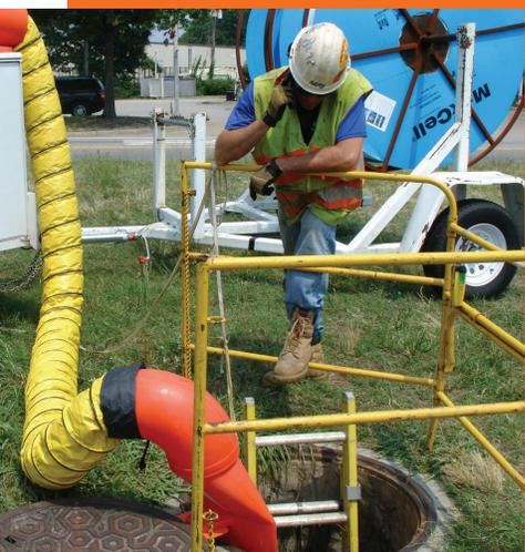
**Rugged, Light Weight, Economical Axial Fans to Provide Fresh Air for Confined Space Ventilation**
