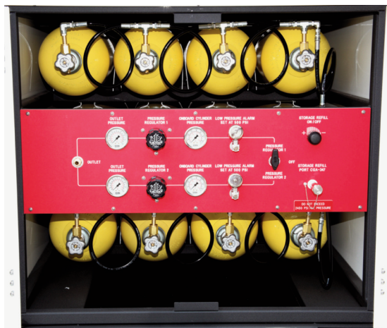
Long Duration Air Storage Hazardous Response Trailers
